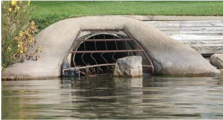
Point Source – look for a pipe bringing water directly to the lake. This pipe could be directing stormwater, gray water, or other water sources to the lake.
